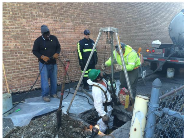
10.2015 Abandonment-in- place for a 5000- gallon Underground Storage Tank (UST) from the 1950s
